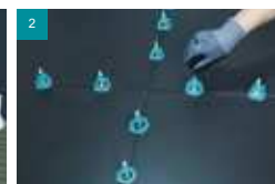
Apply the level washer and level cap to the level base
