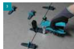
Use the plier to tighten to the required level
