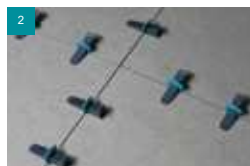
Insert the reusable wedge into each level base
