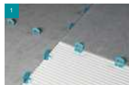
Place the level base under the tiles 10cm from either end
