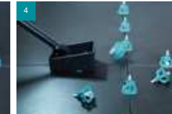
Remove the cap with BIHUI levelling dozer for reuse
